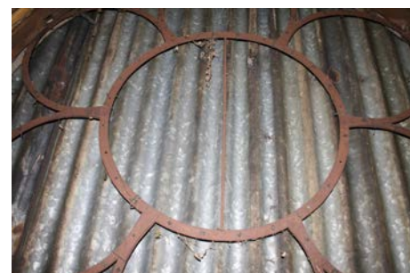
The surviving iron 'rose' window of the 'tin tabernacle' © Pre Construct Archaeology
