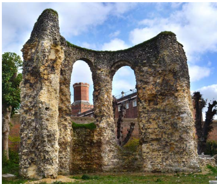
Restored Abbey ruin with sedum turf capping. Reading gaol in the background © Reading Museum
